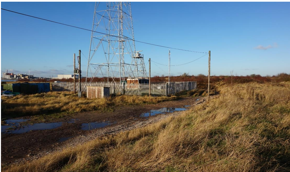
Figure 3: (Image looks toward the north-north-east) The Gravesend-Broadness AWS enclosure at the northern tip of the Swanscombe Peninsula, bordered by steel fencing, radar masts operated by the PLA are also present within the enclosure. A Stevenson screen and 10m wind measuring mast are in the south-east corner of the enclosure (taken by the author).
